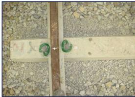
Figure 2. Artificially introduced ballast damage under the left side of the concrete sleeper, (Lam et al., 2012)
