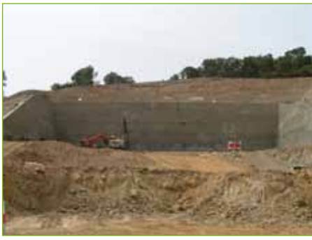
Tunnel Perthus. © D. Allagnat - Egis
