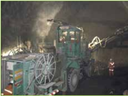
A40, tunnel de Chamoise. © J. Peltier - Scetauroute
